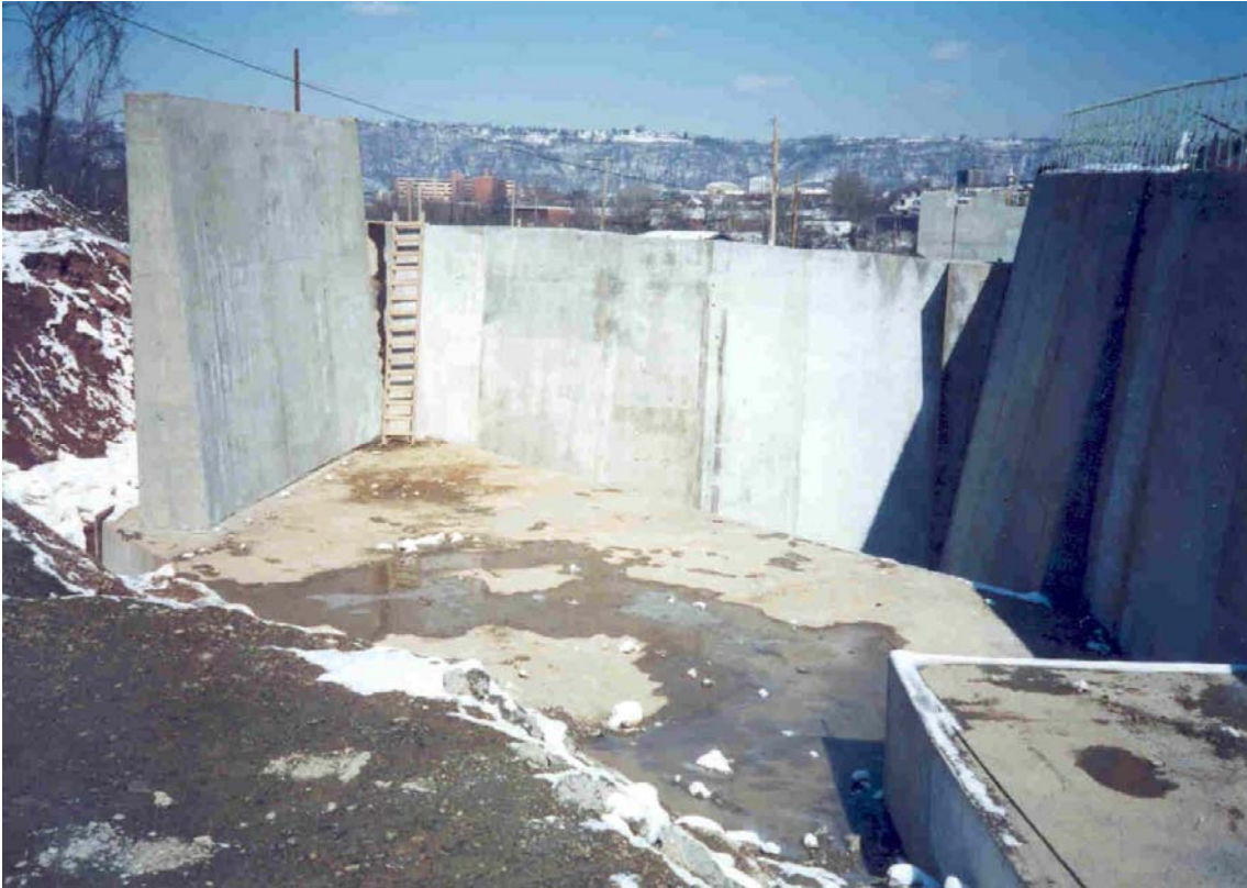
Figure 10-18. CIP abutment with integral wingwalls
